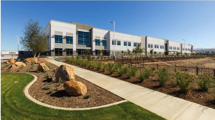
Watson Land Company, developer, owner, and manager of industrial properties, counts more than 23 million square feet of warehouse and distribution facilities throughout the South Bay of Los Angeles, the Inland Empire, and the East Coast.
